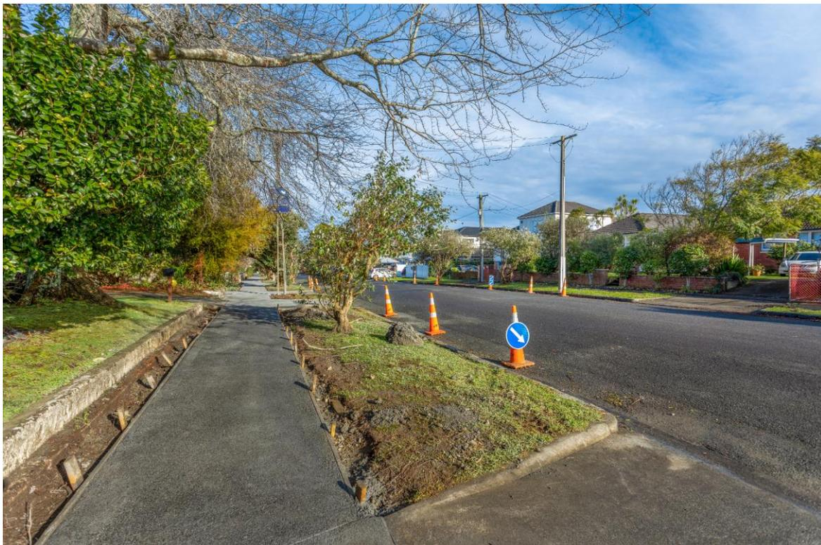
These images are of progress on the large scale Mt Albert Undergrounding Project. The photos show new footpaths that have been reinstated over top of the new underground electricity networks laid in the street. Houses are being systematically connected to these new underground cables, and when they are all connected the old overhead lines and poles will be decommissioned and removed.
